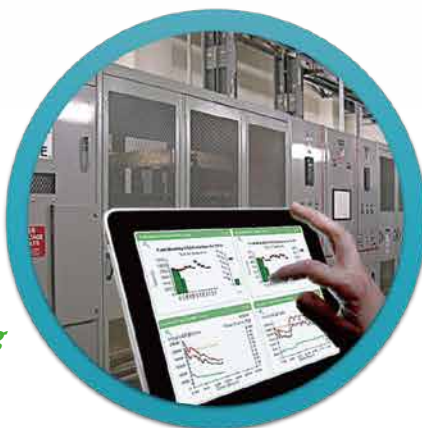
Power Quality Monitoring
